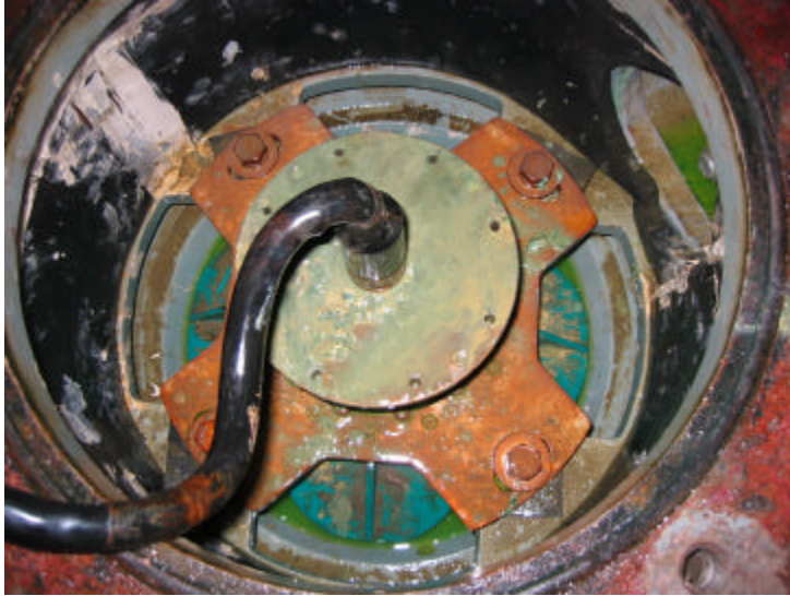
Fig. 1: Top view of the 153-kHz ADCP transducer unit after the well is drained of most of its (light green) anti-freeze fluid. Note the rubber washers (black) below the rust-red mounting plate with 4 mounting bolts.
